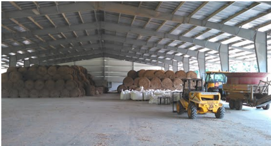
FDC Enterprises, perennial grass biomass processing facility near Fort Pickett, Virginia.
